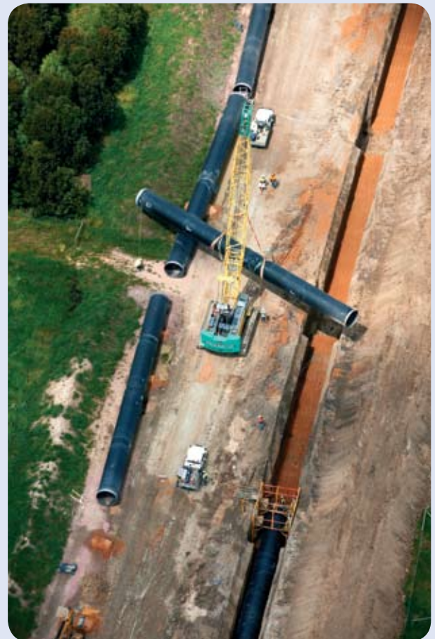
Hydrotesting provides final verification that the pipeline is fit for operation.
